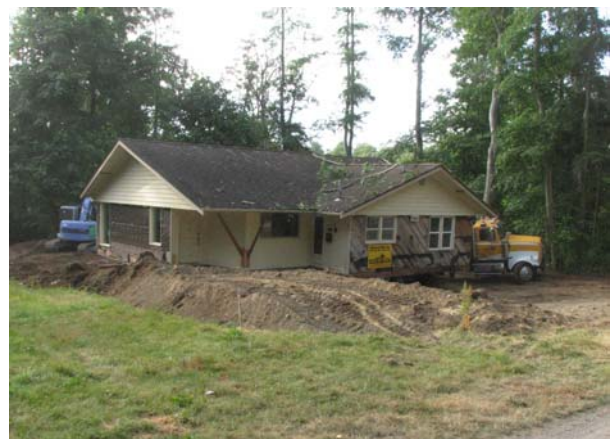
12. In its foundation hole
