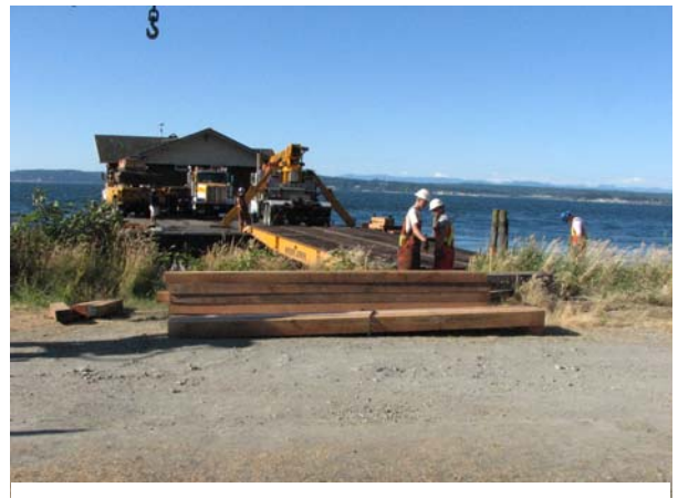
4. Build a ramp ashore
