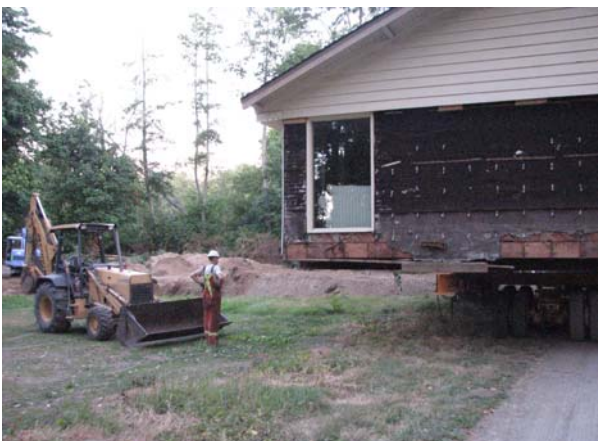
11. Arrival at home site with foundation pre-dug
