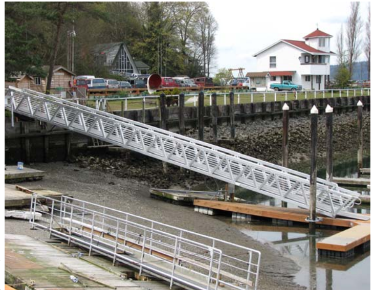
New south gangway shown at a -2.5' low tide, no more climbing Mt. Everest at low tide! Obviously we still need to dredge!
