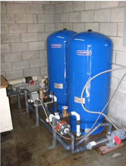
G Tank after repair
